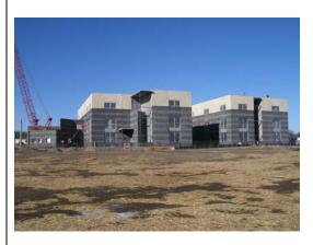
ERA provided the precast structural design for the new **Nova Classical Academy** in **Saint Paul, MN**. The three level, 70,000 square foot charter school includes a classroom wing structured with precast beams, columns, wall panels and plank and a gymnasium and common area structured with precast wall panels and steel roof.
