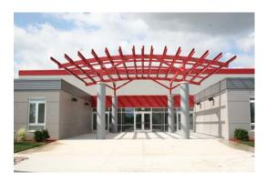
used to reduce the number of pieces which reduced erection time and cost.
