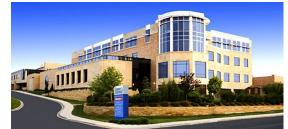
construction utilized Concrete Pan and Joint construction. Stone and brick were used for exterior wall framing with glass curtain wall at the main rotunda.
