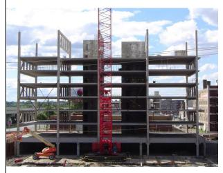
Bookmen Stacks condominiums in Minneapolis, MN utilized the recently patented ER-POST™ precast concrete truss system. The trusses span approximately 70' and are spaced at 40+ o.c. allowing for large bays. Each truss has the ability to support two floors
