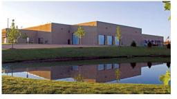
The structure consists of a steel joist/metal deck roof system supported by interior steel beams and columns and perimeter precast concrete bearing walls.
