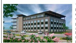
The new 74,000-square foot office building, located in downtown Eau Claire, WI, is a precast structure with steel at the mechanical penthouse. It has four levels, plus a penthouse and a partial basement. The fourth level features an outdoor covered balcony. The building was located
