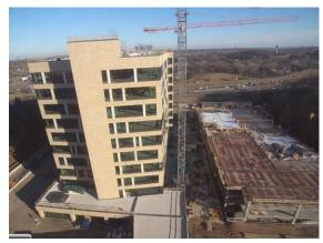
Phase II, building will be 11 stories tall and include 350,000 square feet of office space plus a parking garage with 1,250 stalls. The parking garage will have a total of 8 levels, 5 levels above ground and 3 below ground. An enclosed walkway will connect to the existing building. This was the largest new office building to be constructed in the Twin Cities in 2012.
