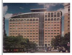
The Lawson Office Building & Parking Ramp, located in downtown St. Paul, is the world headquarters for the Lawson software firm. The building structure is 450,000 sq. ft. with a seven level 1,000 car parking ramp. The 375,000 square foot parking ramp is constructed of post tension concrete, having two levels below grade and five levels above grade with retail at the ground level.
